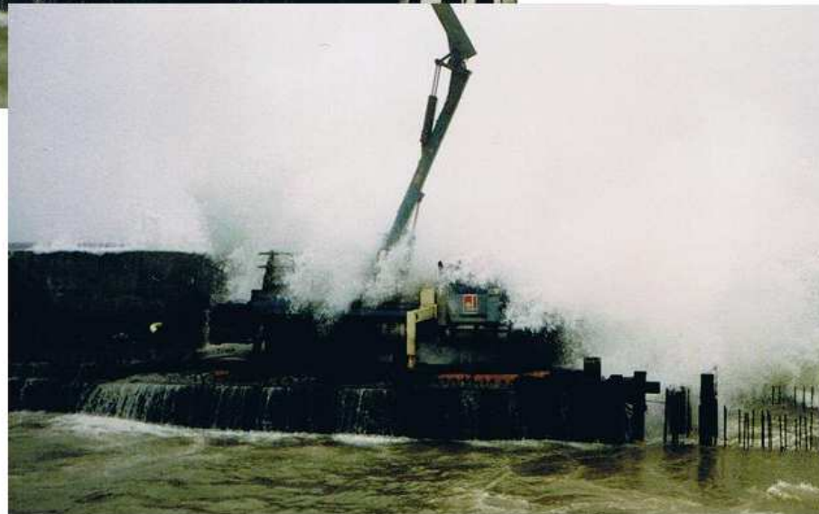
Something Cool: Pumping Concrete, St. Shott's, NL, 1991
